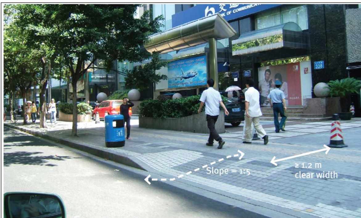
CONSTRUCTION OF FOOTPATHS AT PROPERTY ENTRANCES
